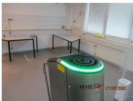
Figure 4: Position of the FLO-D MINI - Mark 2 and the power-humidifier EVA in the test room
